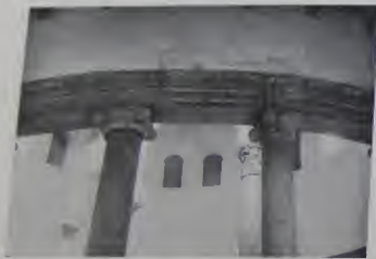
Fig. 162. S. Stefano Rotondo. Elevation of nave showing brick pilasters and arches.
